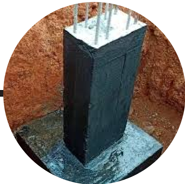
Bitumen coat Footing
